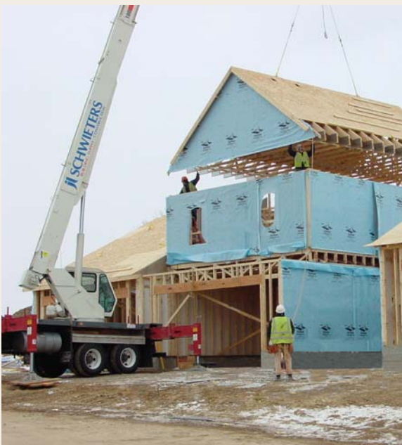
Above left: With wall panels, carpenters can literally build a house in a day. Above right: Schwieters Construction Park is located in Hugo, MN.
